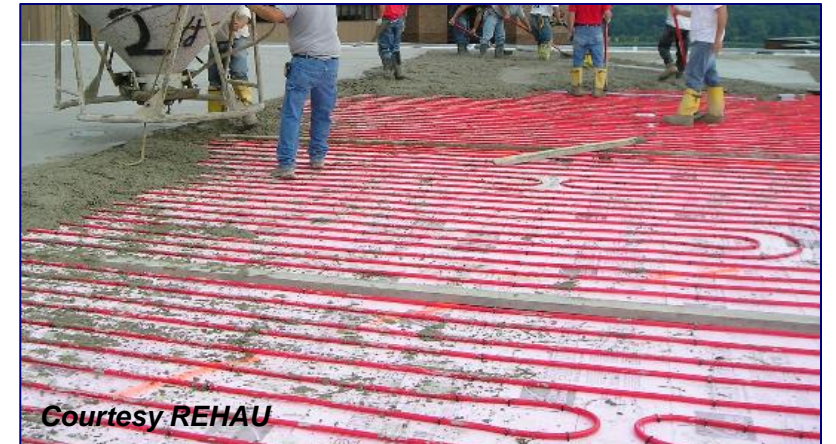
Medivac landing pad on hospital rooftop
