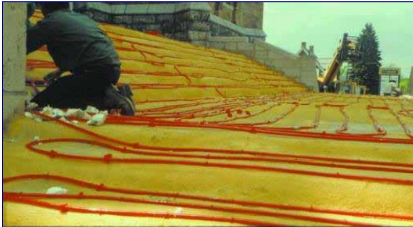
Spray-foam insulation on old stone steps (church)
