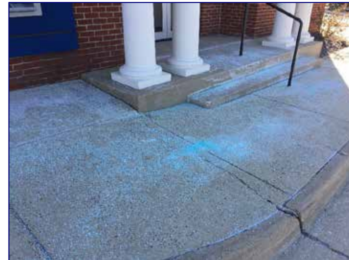
Salt at bank entrance
